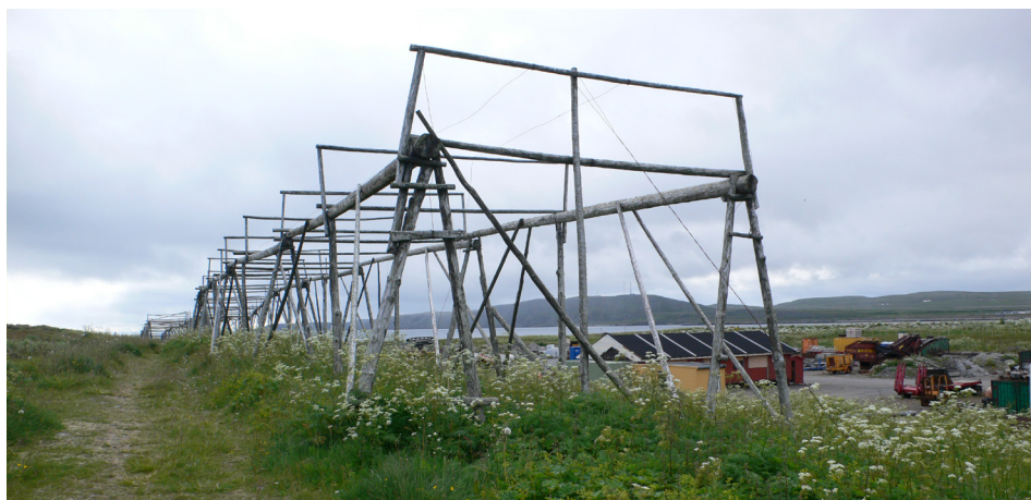
Fig.5. Vardø's structure for drying fish. Photograph: Susana Ventura, 2014.
